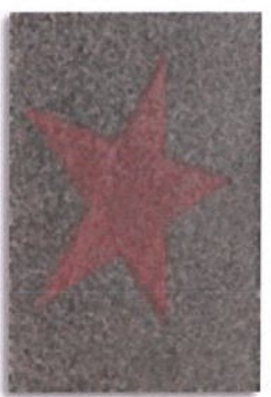
Rubberized surfacing used throughout entire playground for wheelchair accessibility.
